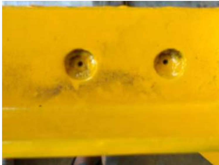
Fig.3 holes drilled over the resistor block for cleaning.
